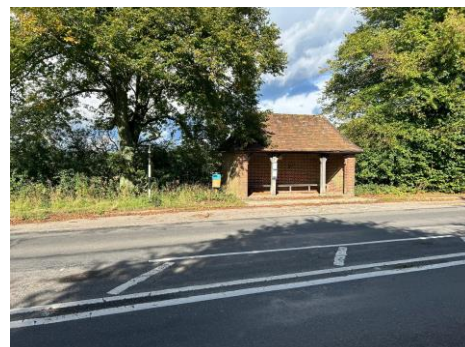
NPC Bus Stop A4130 opp Maker Space
